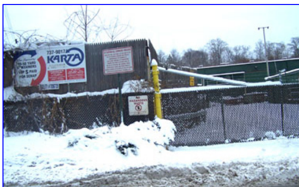
Karta Corporation in the Peekskill Industrial Park, recycled many tons of materials annually and provided employment to many residents of Peekskill and surrounding communities, however their failure to comply with protective regulations led to their closure. Photo by http://ncnlocal.com
